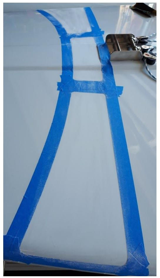
5. Lightly sand the base of the moulding to be glued to the deck.
