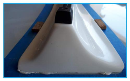
Put weights (e.g. 2 Litre water containers) on top of the track to ensure it is firmly but evenly holding the track down on the deck. If using clamps do not over-tighten them as it may squeeze out too much adhesive. Clean up any excess adhesive with 100% Denatured Alcohol/Methylated Spirits. **Do not use Acetone.**
